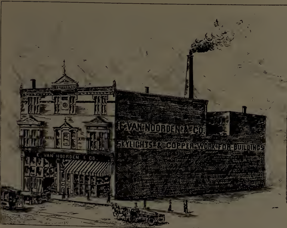
WORKS OF E. VAN NOORDEN & CO., 383 and 385 Harrison Avenue. Metal Roofers, Manufacturers of Copper Work, Cornice Skylights, and Metallic Archi- tectural Work generally. Established 1873. Employ eighty-five hands.
